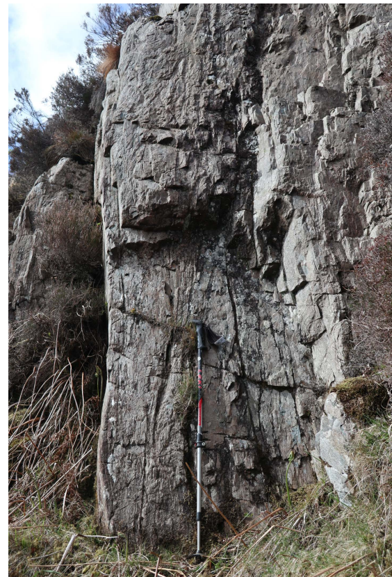
Figure Sleat 2.7: Vertical planar fabric of the mylonite. Pole c. 1m long.
