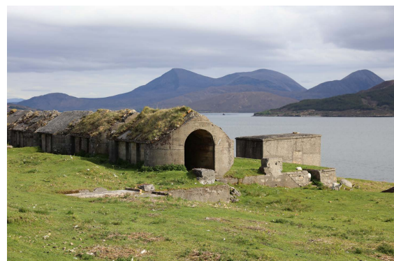
Figure Raasay 6.10: Remnants of the kilns at East Suisnish, used to calcine the ore prior to shipping.
