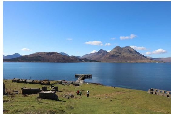
Figure Raasay 6.9: The derelict processing plant above the East Suisnish pier. The row of roofed buildings to the left are the remnants of the kilns (removed when the operation closed in 1919) and the unroofed terrace on the right was offices, stores and workshops for joiners, blacksmiths and engineers.
