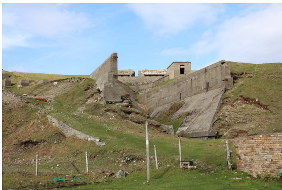
Figure Raasay 6.12: Ore hopper, with remnants of kilns behind, within the processing plant, East Suisnish. View is towards the NE.
