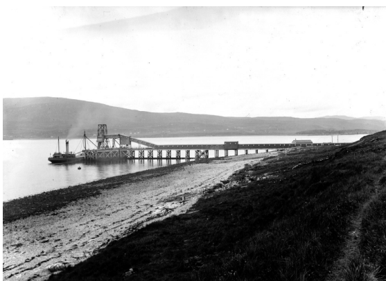
Figure Raasay 6.7: Pier at East Suisnish with conveyor belt and loading elevator. Ore is being loaded onto a ship for transport to the mainland. View is towards the west. [BGS P000046]
