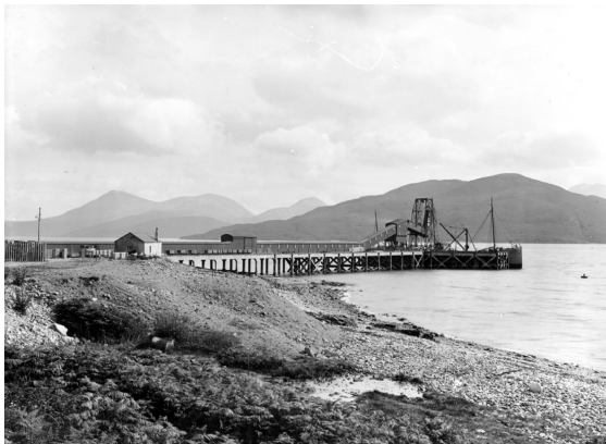
Figure Raasay 6.6: Pier at East Suisnish with conveyor belt and loading elevator. View is towards the SE. [BGS P000045]
