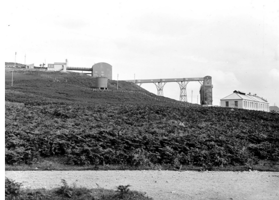
Figure Raasay 6.8: Processing plant at East Suisnish, viewed towards the east. At the top of the short rail incline is the pier hauler incline house, to the right of which is the crusher (arched roof) and conveyor to the top of the kilns. Coal was taken to the crusher via the short rail incline, where it was mixed with the unprocessed ore and thence to the kilns. The white building, to right, comprised offices, stores and workshops for joiners, blacksmiths and engineers. [BGS P000044]
