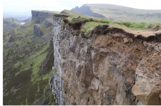
Figure North Skye 9.19: The unstable face of Sròn Vourlinn where it has partially collapsed, exposing relatively fresh lava. Keep well away from this unstable edge.
