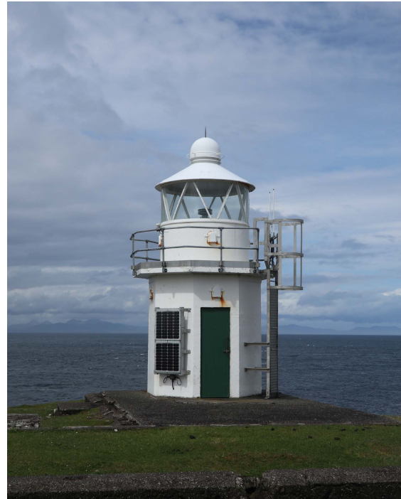
Figure West Skye 4.20: Waternish Point Lighthouse, a wee bobby dazzler of a lighthouse, powered by solar panels, a 1980 replacement of the original 1924 lighthouse designed by David and Charles Stevenson.
