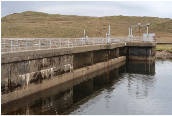
Figure North Skye 2.2: Storr Lochs dam/viaduct.
