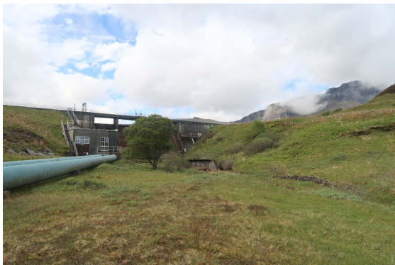
Figure North Skye 2.3: Storr Lochs dam/viaduct.
