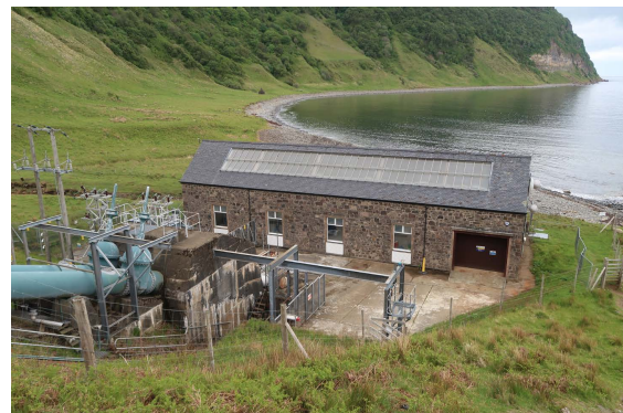
Figure North Skye 2.8: Generator house of the Storr Lochs hydroelectric scheme.
