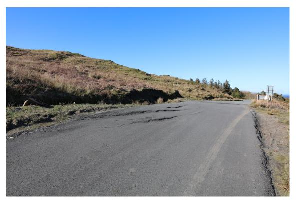
Figure 10-47 – Road damage at Flodigarry. Repairs are made on an almost annual basis due to ongoing minor movements within the landslipped material as it migrates eastwards towards the coast.
