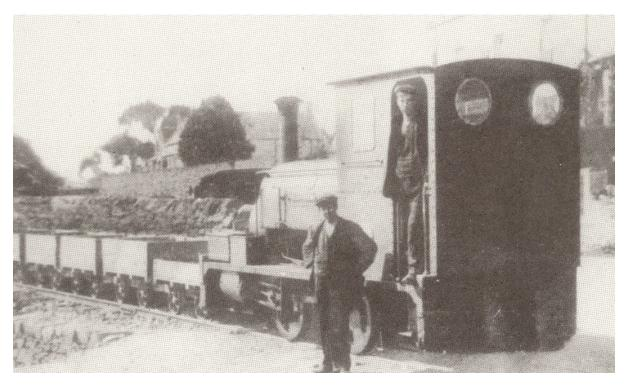
Figure 11-4 – The steam locomotive *Skylark*, used to haul material from the Kilchrist quarries to the pier at Broadford.
