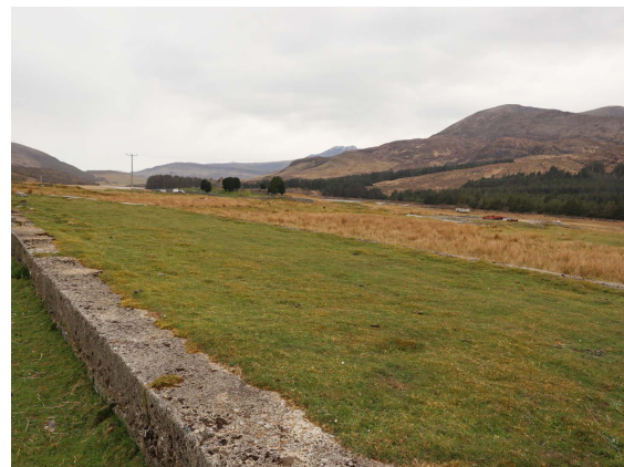
Figure Strath 3.20: Loading platform at the processing plant building, immediately south of the Broadford-Elgol (B8083) road at [NG 6198 2074] .
