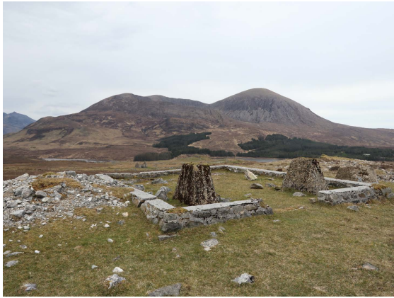
Figure Strath 3.16: Part of the quarry building infrastructure (crusher?) at [NG 6185 1979] .
