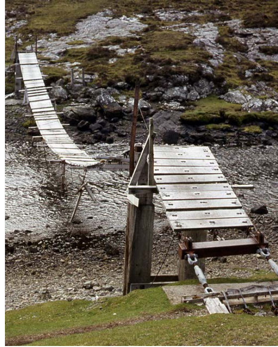
The footbridge at Camasunary, May 1983 © Ian Taylor.
