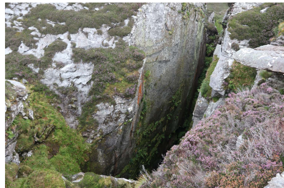
Figure Raasay 5.40: Detail of major NW-SE -trending fissure within the Beinn na Leac landslip. Fissure depth is in excess of 20m.
