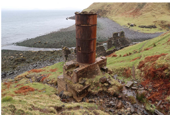
Figure North Skye 4.11: Remains of diatomite processing plant at Inver Tote. The brick structure with chimney was a kiln used to calcine (heat treat, driving off CO 2 ) the diatomite and the stone building beyond was a drying shed.
