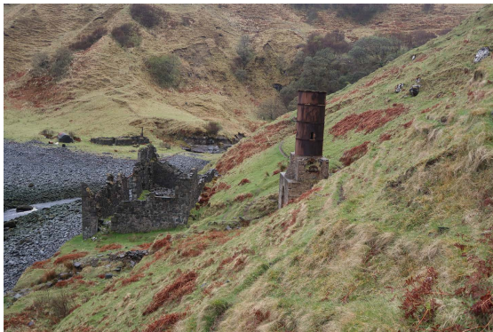
Figure North Skye 4.10: Remains of diatomite processing plant at Inver Tote. The brick structure with chimney was a kiln used to calcine (heat treat, driving off CO 2 ) the diatomite and the stone building beyond was a drying shed.
