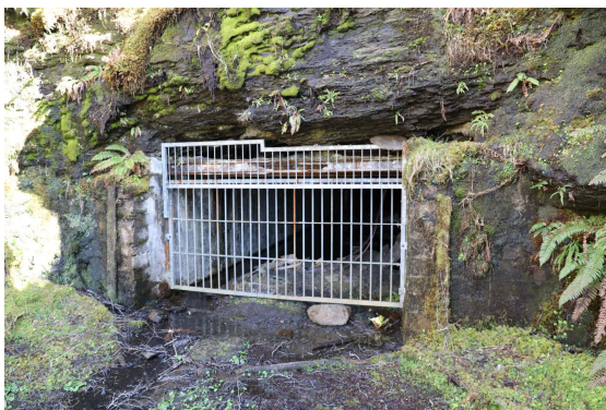
Figure Raasay 4.22: Mine #1 entrance.
