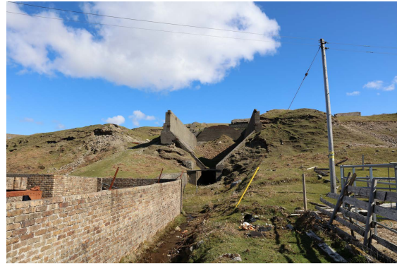
Figure Raasay 4.47: Processed ore hopper within the processing plant, East Suisnish. View is towards the NE.
