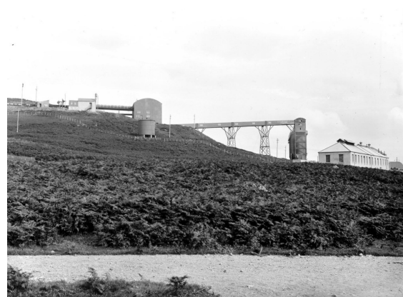
Figure Raasay 4.40: Processing plant at East Suisnish, viewed towards the east. At the top of the short rail incline is the pier hauler incline house, to the right of which is the crusher (arched roof) and conveyor to the top of the kilns. Coal was taken to the crusher via the short rail incline, where it was mixed with the unprocessed ore and thence into the kilns. The white building, to right, comprised offices, stores and workshops for joiners, blacksmiths and engineers. [BGS P000044]
