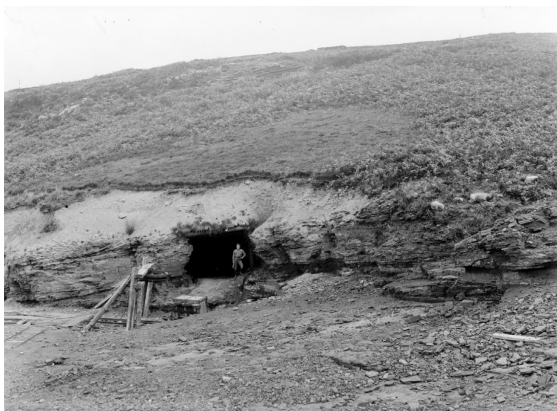
Figure Raasay 4.8: Trial adit into the Raasay Ironstone Formation located at the top of the incline in the area where opencast production occurred. Note rail head. Person for scale. [BGS P000039]
