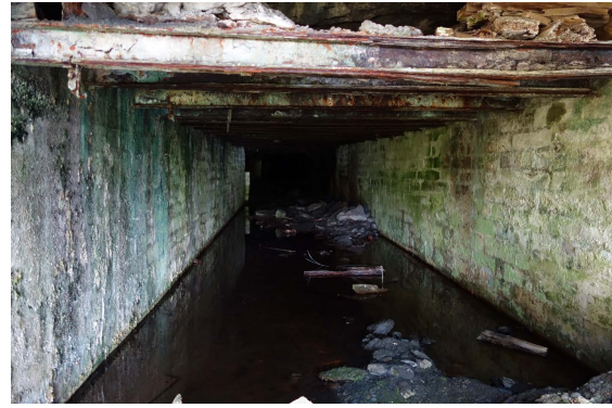
Figure Raasay 4.23: Partially flooded Mine #1 adit, leading to a network of (reputedly) 8km of tunnels from which the ore was removed.
