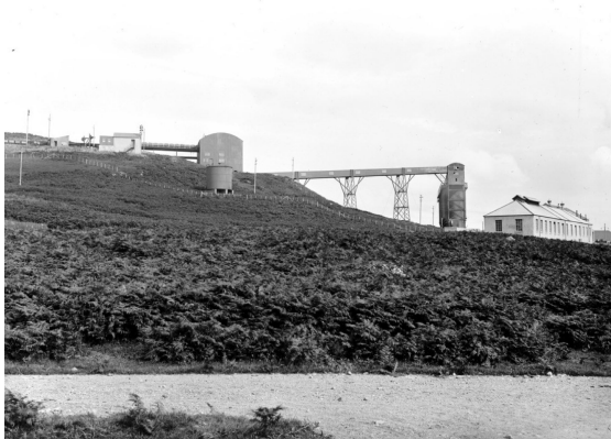
Figure Raasay 4.11: Processing plant at East Suisnish, viewed towards the east. At the top of the short rail incline is the pier hauler incline house, to the right of which is the crusher (arched roof) and conveyor to the top of the kilns. Coal was taken to the crusher via the short rail incline, where it was mixed with the unprocessed ore and thence into the kilns. The white building, to right, comprises offices, stores and workshops for joiners, blacksmiths and engineers. [BGS P000044]
