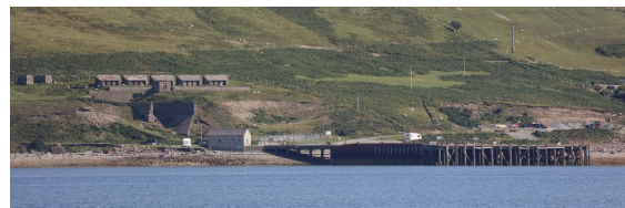
Figure Raasay 4.48: The East Suisnish pier, and the main processed ore hopper and kilns of the processing plant.
