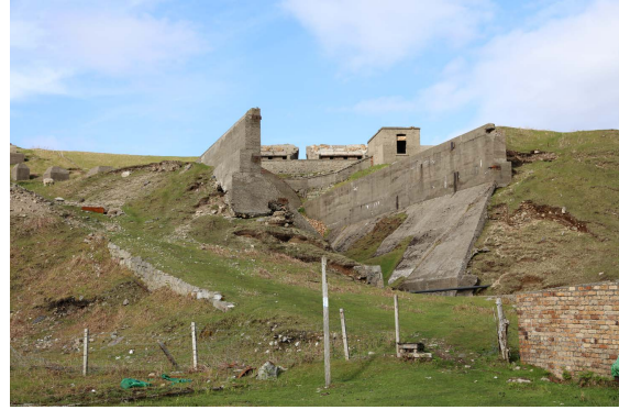
Figure Raasay 4.46: Processed ore hopper within the processing plant, East Suisnish. View is towards the NE.
