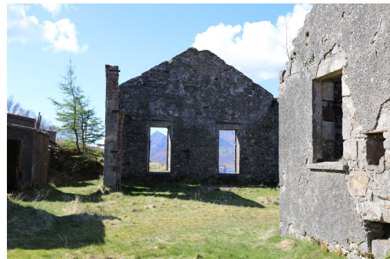
Figure Raasay 4.24: Derelict main hauler house (nearest) and compressor house, close to the entrance to Mine #1. The hauler house contained the winding gear used for the cable haulage system.
