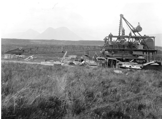
Figure Raasay 4.12: A Bucyrus Steam Dragline ('Steam Navy') near to the entrance to Mine #1, used to remove superficial material from the area developed for opencast extraction. [BGS P000047]
