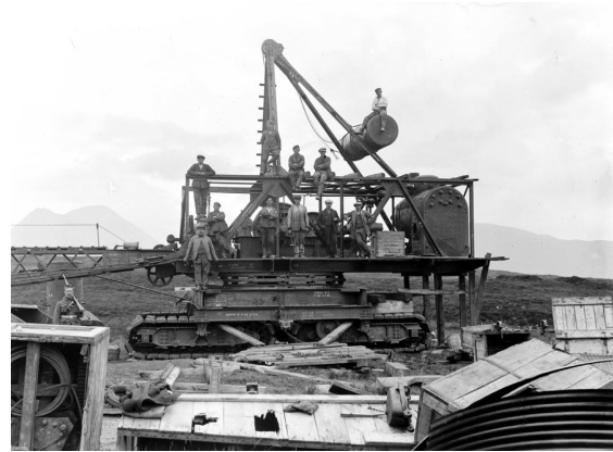
Figure Raasay 4.13: Detail of Bucyrus Steam Dragline ('Steam Navy') near to the entrance to Mine #1, used to remove superficial material from the area developed for opencast extraction. Note armed guard, suggesting that at least some of the workers perched on the dragline are German prisoners-of-war. [BGS P000048]
