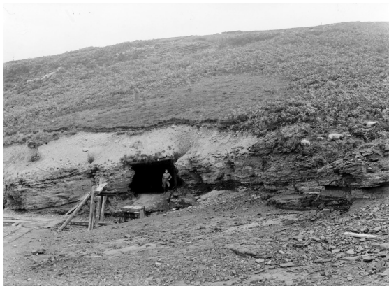
Figure Raasay 4.28: Trial adit into the Raasay Ironstone Formation located at the top of the incline in the area where opencast production occurred. Note rail head. Person for scale. [BGS P000039]
