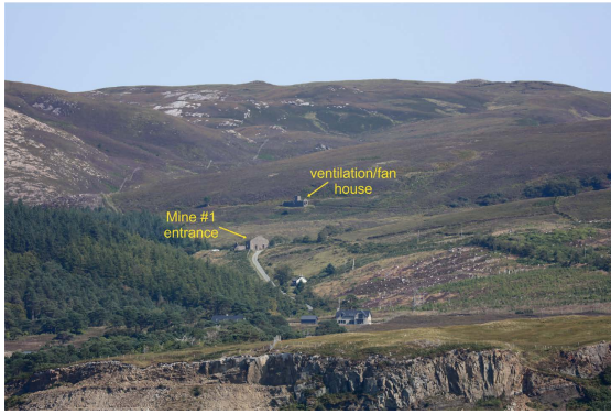
Figure Raasay 4.20: Derelict buildings at entrance to Mine #1 (right of centre in the middle ground) and beyond, the ventilation (fan) house. View is towards the NE.
