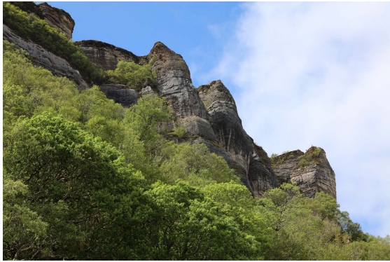
Figure Raasay 2.16: Fissures within the cliffs, leading to the formation of (unstable) rock pillars, Creag na Bruaich. View is towards the NW.
